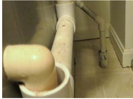
Drain Hole in floor ^
